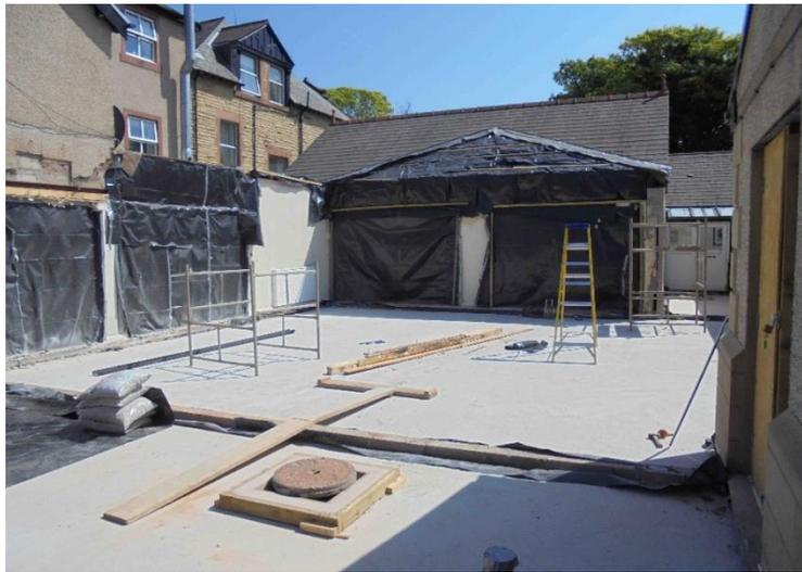
**The photos show where half of the old dining room use to be. The concrete was poured into the area in readiness for the timber walls and roof to be constructed. We recently sought guidance from firms about the internal design, to ensure the lighting and contrast are suitable for visually impaired people and the layout was right for people who have dementia.**
